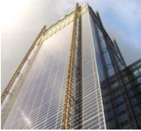
Resim 6. The CIS Tower - Manchester, UK
